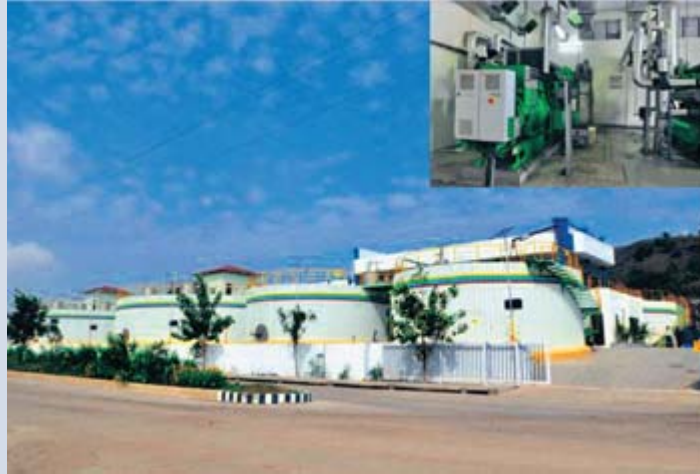
1.4 MW Power Project based on mixed industrial wastes at Jalgaon (inset Bio-gas engines)
