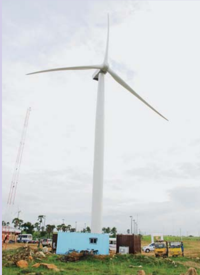
2 MW R&D Wind Turbine at Kayathar, Tamil Nadu
