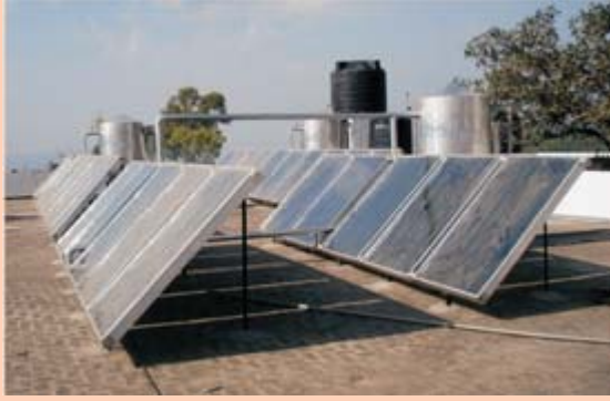
Solar Water Heating System at Vaishnodevi, Katra, under Special Area Demonstration Project Programme
