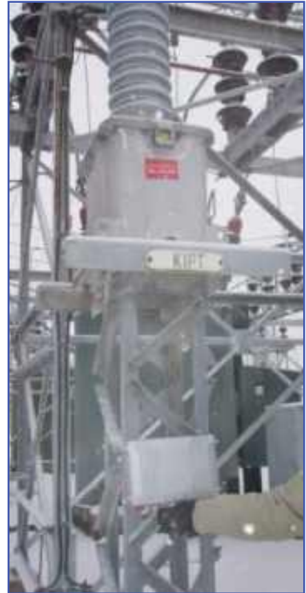
External, on a structure
